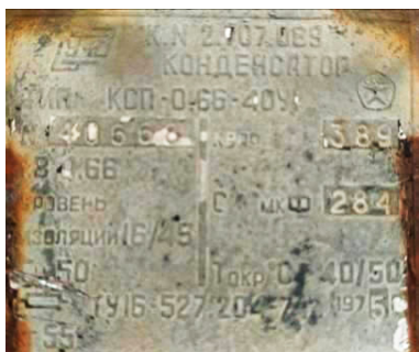
Figure: 12. Nameplates of capacitors type КСП-0,66-40У1
